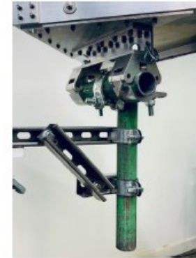
Reflector fitted to mount using the Doughty Half Couplers
