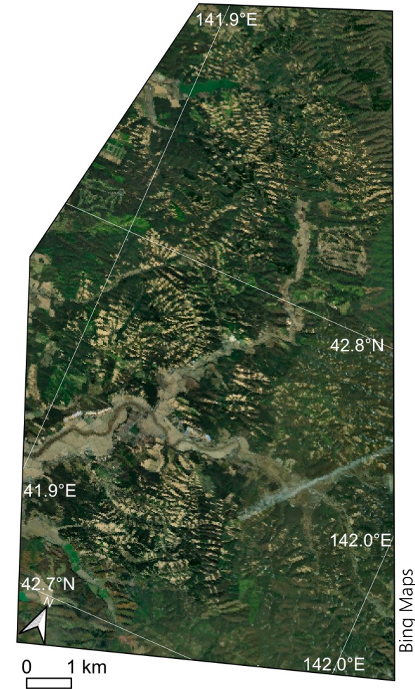
Landslides due to 2018 Hokkaido Eastern Iburi earthquake and typhoon
